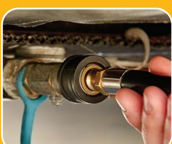
INSERT QUICK CONNECT MALE ADAPTER DIRECTLY INTO FUEL SOURCE
